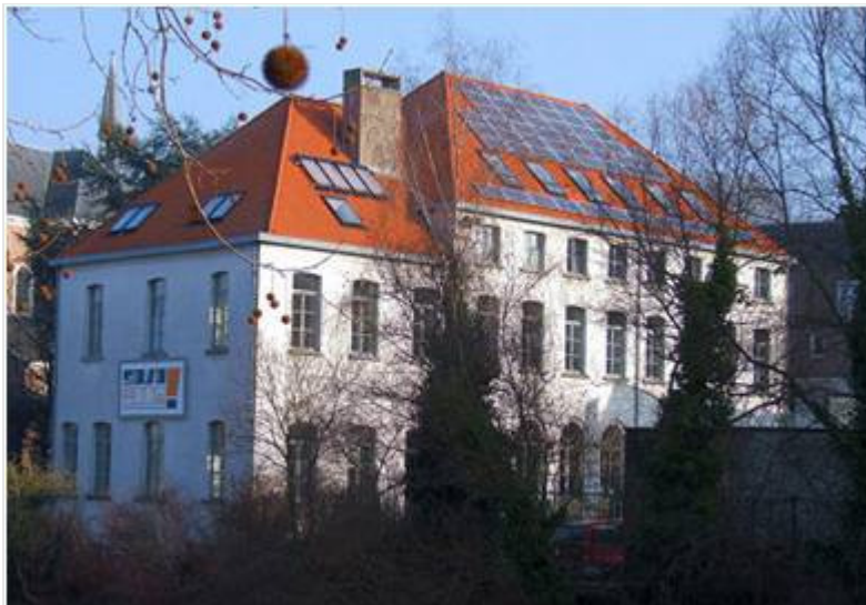
Photo 1. Not uncommon in Belgium: PV modules on old building in Gent.
